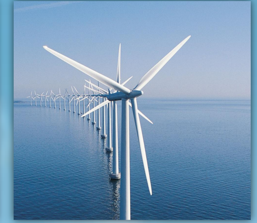
2008, Offshore 2.5MW turbines [5]
