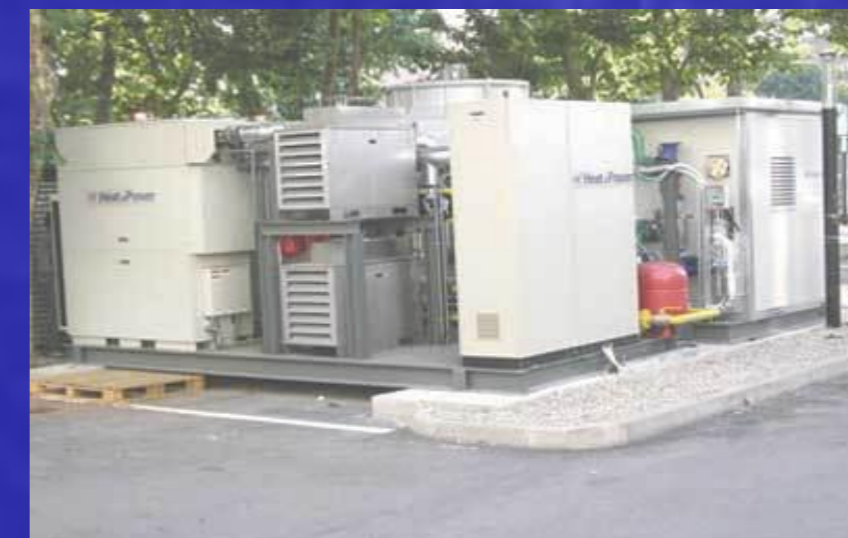
Figure 1. CHP offers a significant decrease in electric power system load especially during hot summer months. CHP advantages, in comparison with conventional cooling devices, are non-emission of harmful freons into the atmosphere and utilization of rejected heat produced in cogeneration facilities. However, CHP is not used only for facility heating and cooling, but also for industrial processes demanding lower temperatures.
