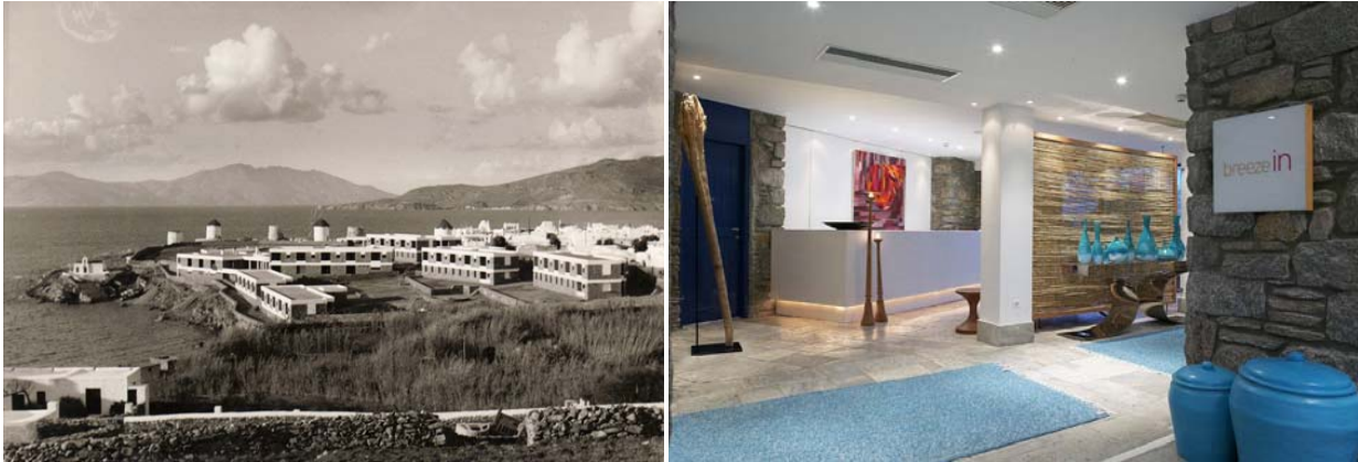
Figure 5,6: Xenia of Mykonos, architect A. Konstantinidis. left-General view (1960) , source: Konstantinidis A (1981), Projects + buildings, A. Konstantinidis, Athens: Agra Ed. and A. Konstantinidis, pp.218. Right- Inside, current situation, source: hotel's site.
