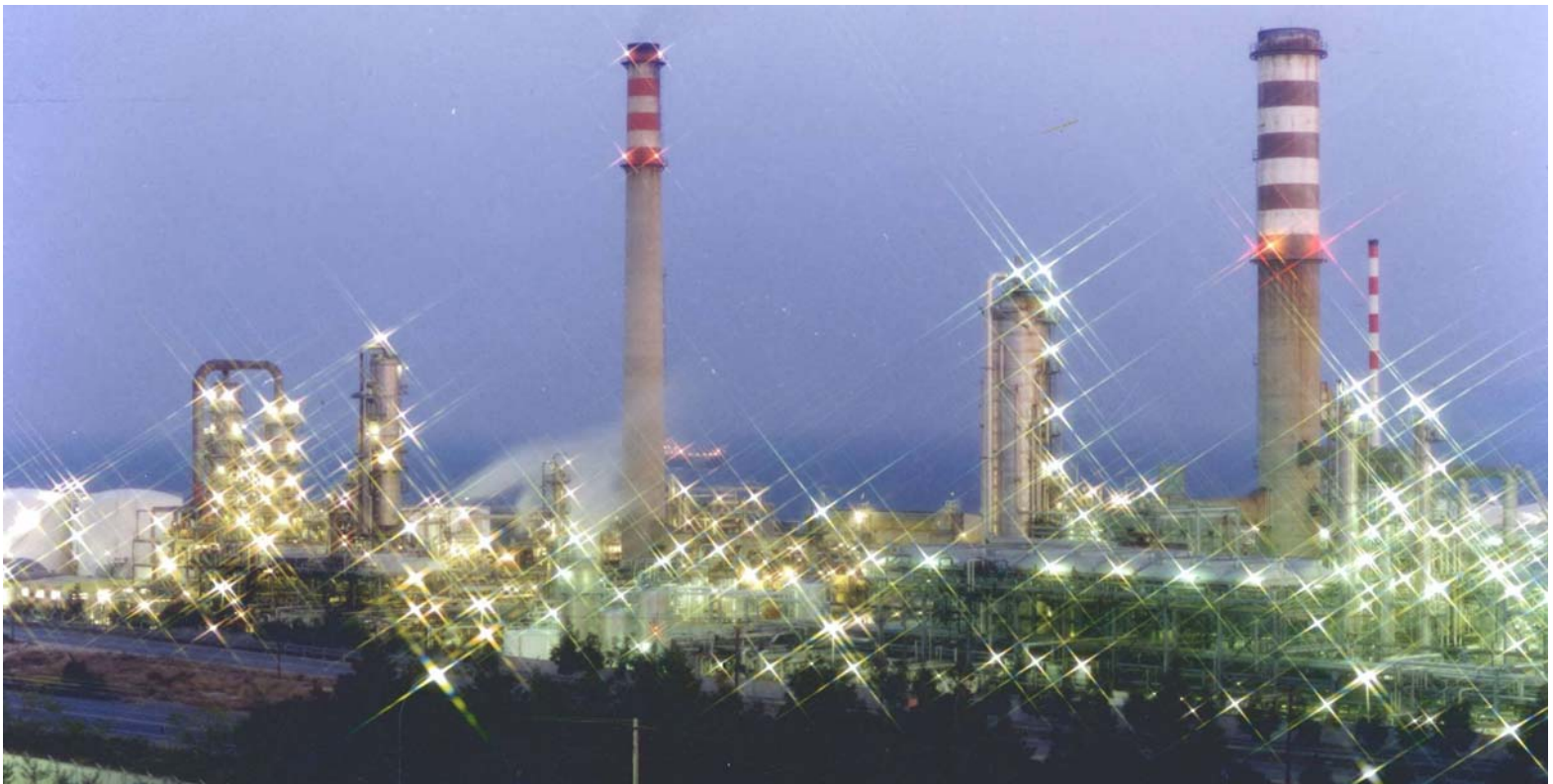
Motor Oil Hellas Refinery
