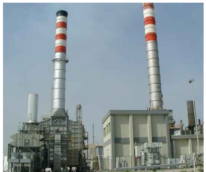
Motor Oil Hellas Refinery Steam & Power Congeneration
